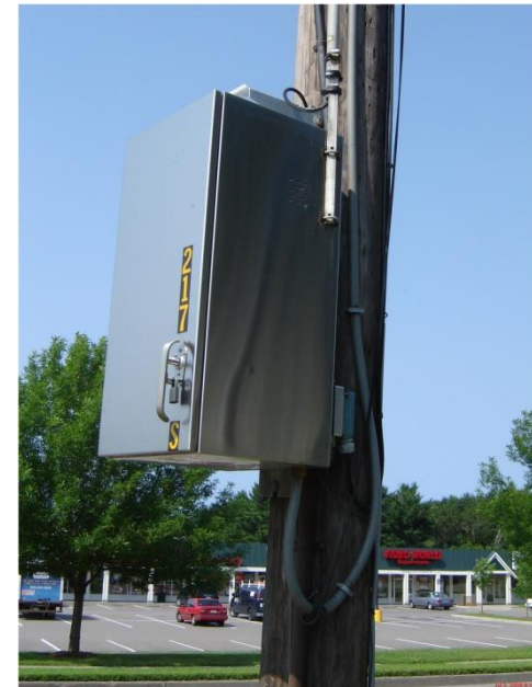
S&C Scada Mate Switch A1 Controller
